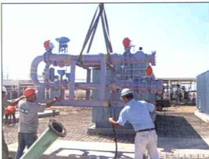
AFC™ being lowered into place in Maipo, Chile
