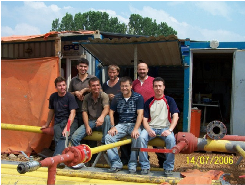
Top: Close-up of Gas Regulation prior to Blender Bottom: Our on site team at Ford (Turkey) site.
