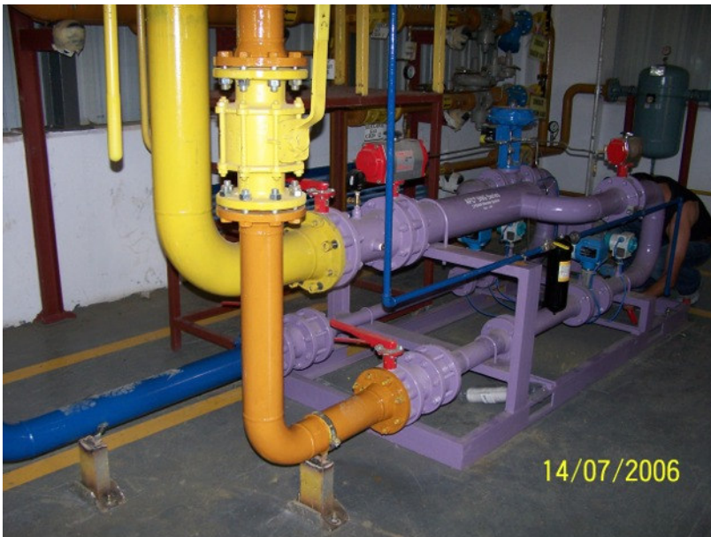
(1) AFC™ Blender at 180MMBTU/h and 1.75 bar g SNG
