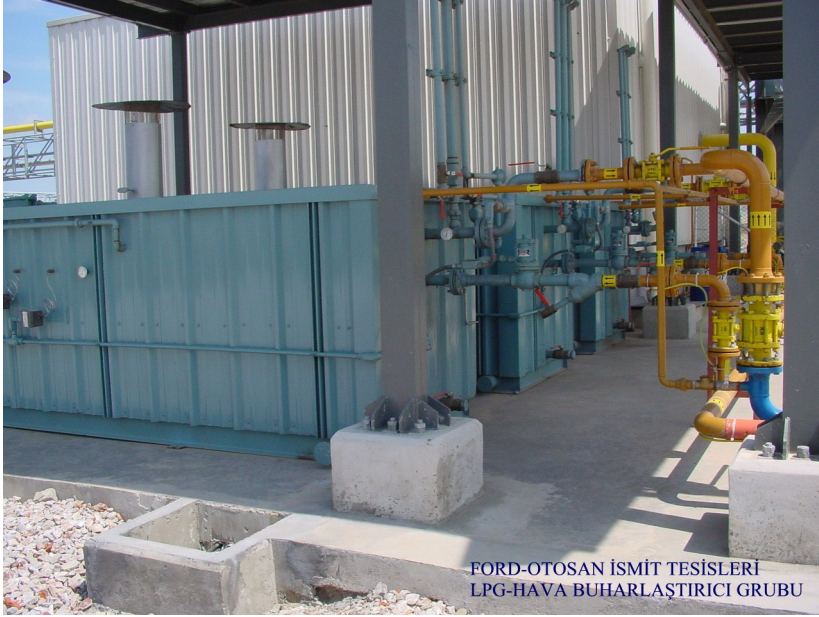
Close-up of AQUA-GAS® Vaporizers
